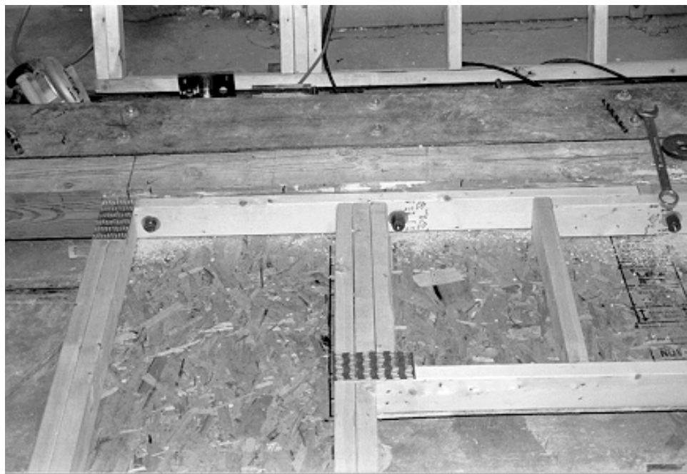
Figure 3 Close Up of Corner Framing and Anchor Bolt (Wall 6)
