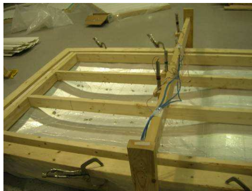
Figure 9. Negative system failure where sheathing failed after siding failed
